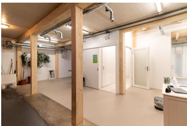
Structure poteaux-poutres centrale
