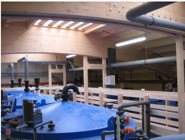
Hall de stockage zone 1
